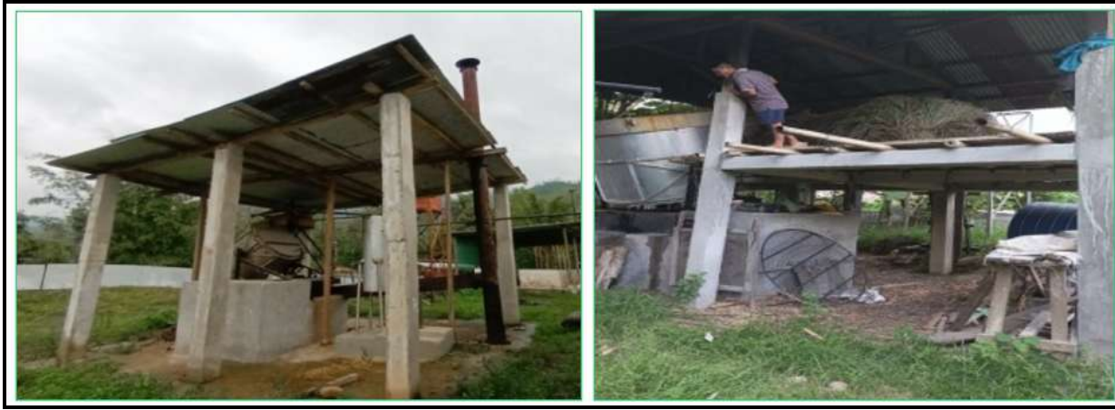
One ton capacity hydro-steam distillation unit established at Seram Village, East-Siang district, Arunachal Pradesh
